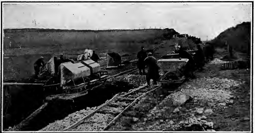
IN NORTHERN FRANCE. French Sappers constructing a railway.
